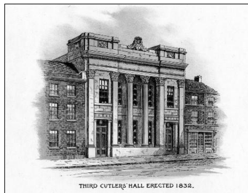
The Cutlers' Hall Source: Picture Sheffield
