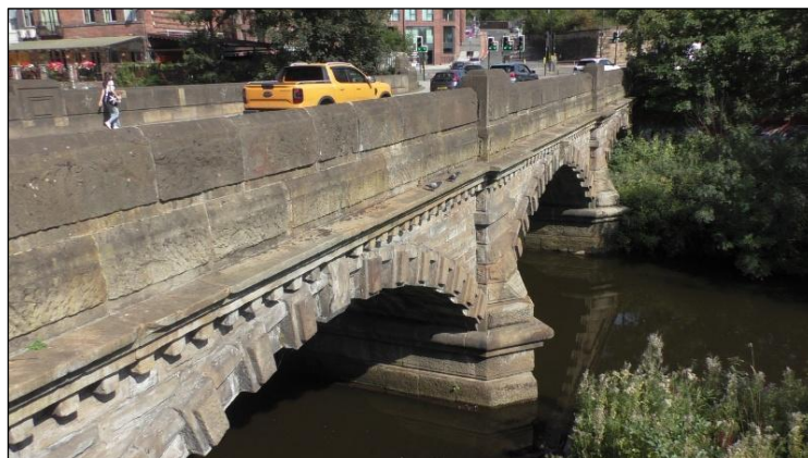
Borough Bridge Source: David Worth
