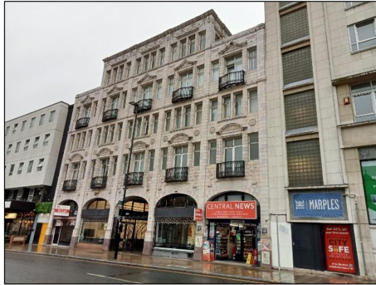
The White Building, Fitzalan Square Source: SGCT Archive
